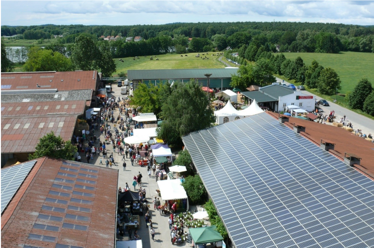
Photo 9: Array of roof-mounted photovoltaic panels
